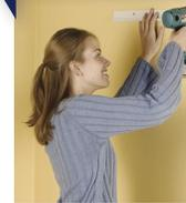
Install rail at desired height using #12 x 2 1/2" screws and drywall anchors provided (88" is standard height measured from top of rail). Use 1/8" bit to drill pilot holes for screws going into studs, and use 1/4" bit to drill holes for drywall anchors.
