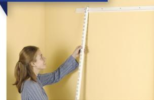
Hang uprights from the rail, spaced no more than 32" apart. Drill holes for stud or wall anchors and secure each upright in two locations using #10 x 2" or #12 x 2 1/2" screws (both size screws work with wall anchor).
